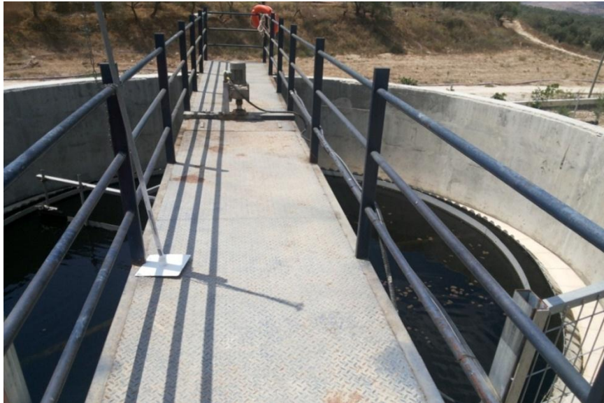
Figure 5: Secondary Settling (sedimentation) Tank at AWWTP.
