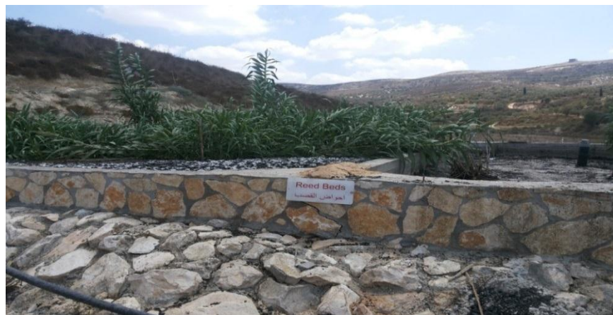
Figure 7: Reed Beds in AWWTP.
