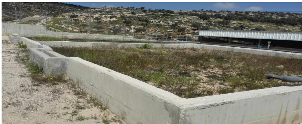
Figure 14: Drying Beds at TRWWTP.
